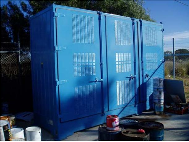
**Plate 37: Typical HHW Storage Locker**
