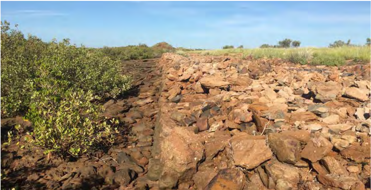
Figure 8. Photograph of Adhoc Rock Protection South West of Cossack Townsite
