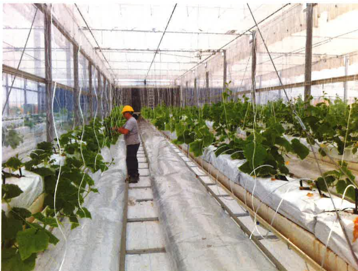
Greenhouse in Qatar. The air is introduced at the far end and distributed down the greenhouse in polythene ducts. The air is extracted at the other end behind the photograph. Here the shade screen is pulled closed to protect the young plants. The irrigation lines are inserted next to the plants in the coir slabs.
