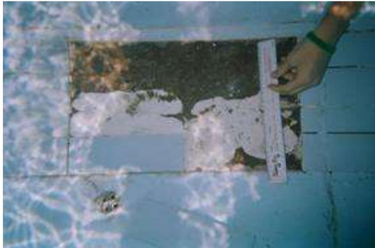
1.15M EXPANSION JOINT – FAILED SEALANT
