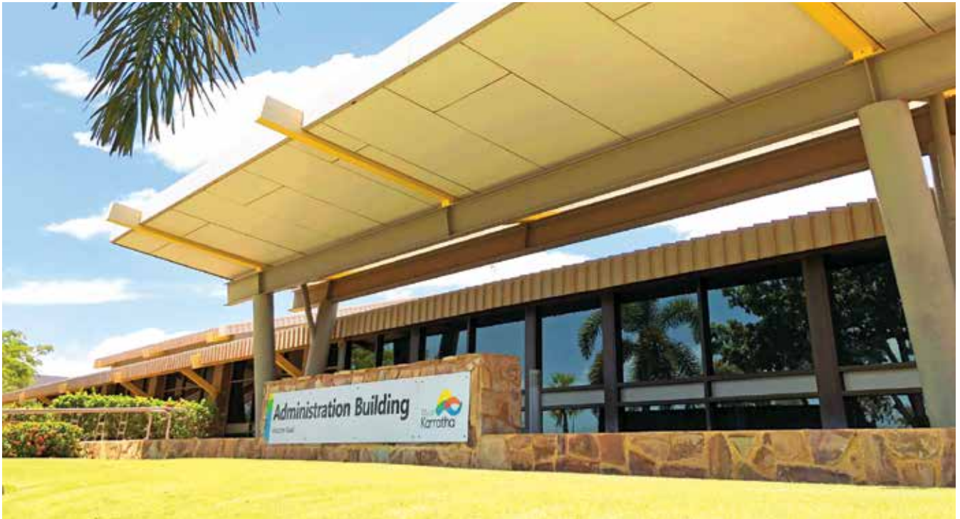
City of Karratha Administration Centre
