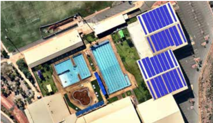
Completed works on the $1.58m Karratha Leisureplex Solar Initiative.
