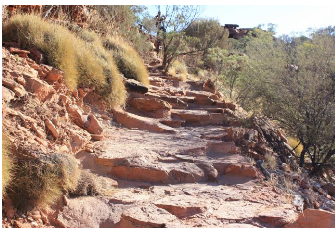
Above: rock steps need to be constructed to look as natural as possible while fulfilling their intended function which is to make steep ascents/descents as safe as possible and providing a firm stable footing.
