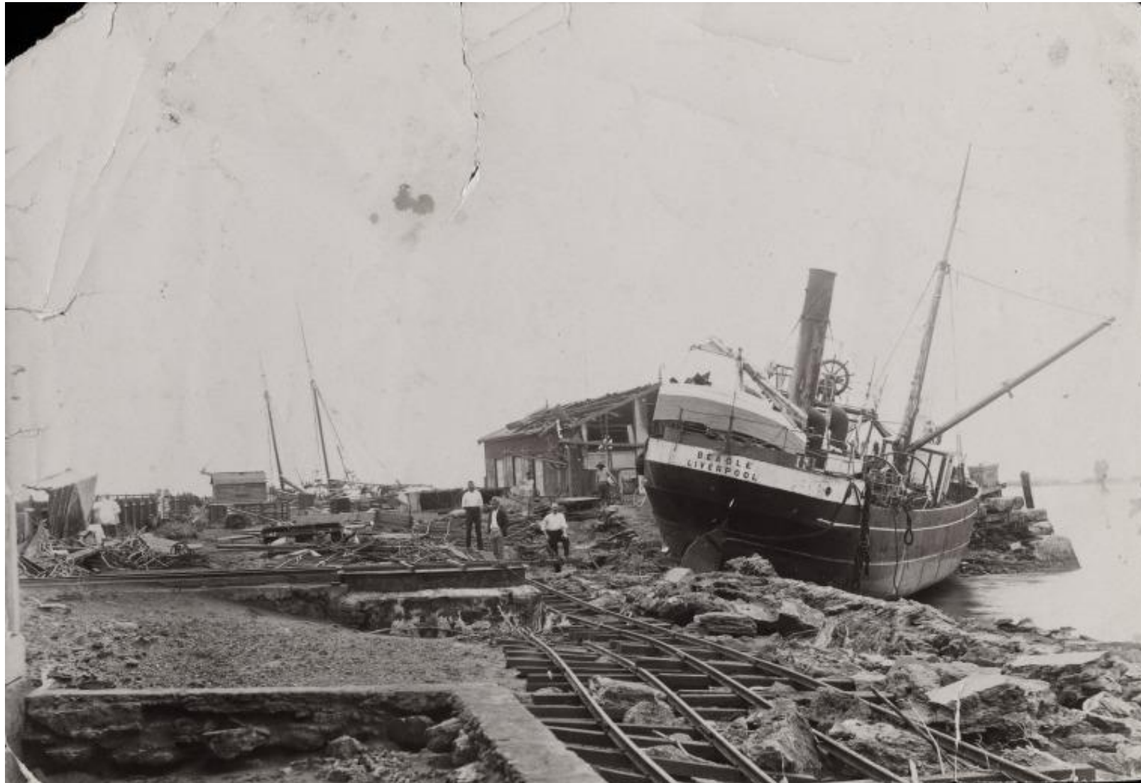
Cyclone damage at Cossack Wharf, with the schooner Harriet and steamship Beagle washed ashore, 1898.
